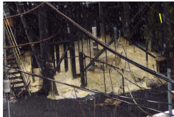
No. 1 Intake Shaft Seal Repairs
