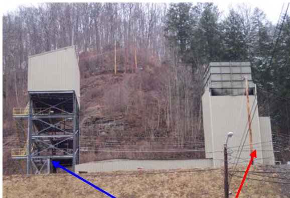
No. 8 Shaft Intake & Return
