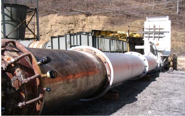
Tubes connected at No. 9 Shaft
