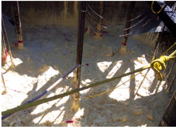
Service Shaft (9 feet below ground level)
