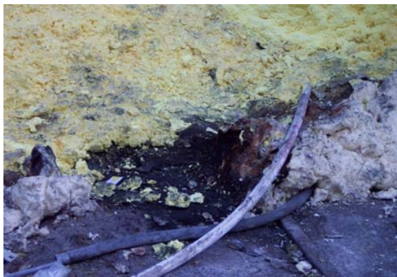
Observed poor application at No 8
