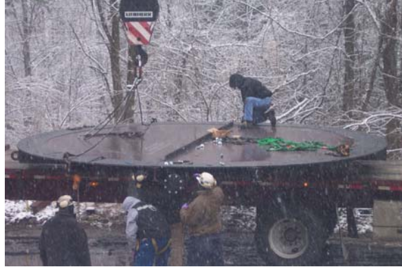
Joining of No. 9 Shaft Seal
