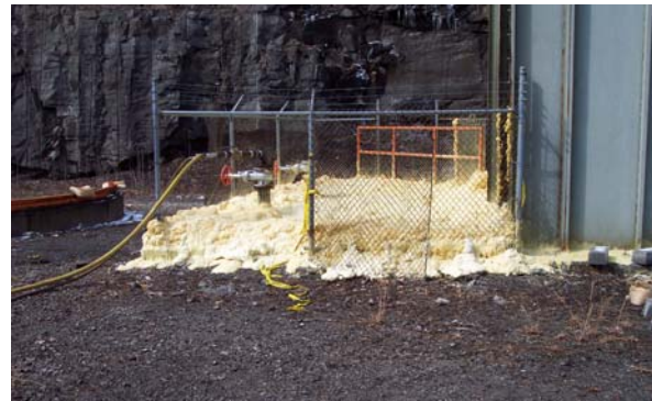
Mine portal seal utilizing PUR Note: Yellow Nitrogen hose
