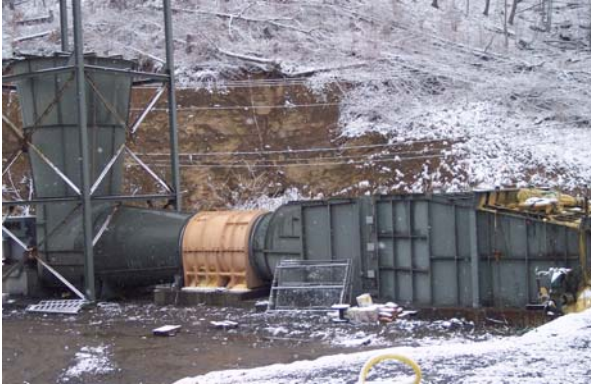
No. 9 Shaft Return Side
