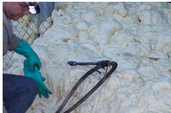
Close inspection prior to sealing
