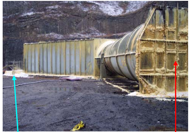
RokLok 70 coating at No. 2 Intake & Return
