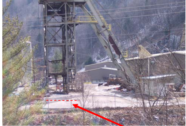
Service Shaft (approximate seal level)
